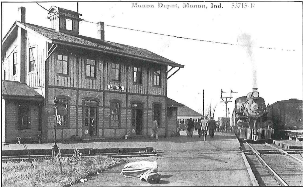
This two-story frame depot at Monon was an 1893 expansion of the single-story depot depicted on page 33. The K-2-class 4-6-2 eased up to the platform was built by Brooks in 1906. In 1916, this station would be replaced by a limestone structure. (DAVE FERGUSON'S PHOTO ART)
