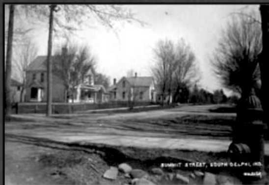
Left: Summit Street 1908. Right: Working on S. Washington St. in 1908. The brick house on the left is 104 W. North, and the single story house in the middle is 101 W. North (Dr. Seese's office).
