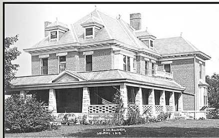
Edward built "The Bowen House" at 100 Riley Road in 1900
